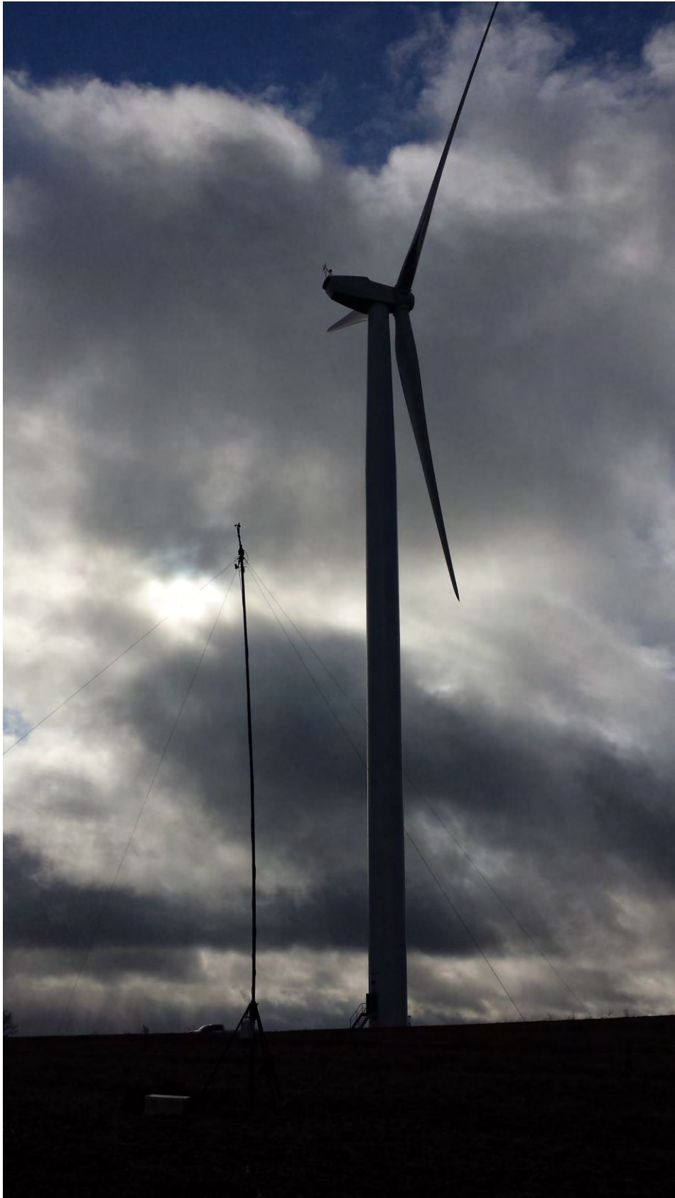
Photo 2: Photo from the wind met mast towards the turbine
