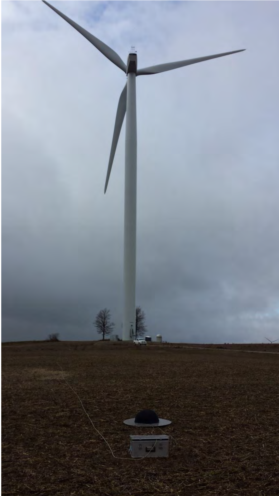
Photo 1: Photo of the microphone and board towards the measured turbine of the type Servion MM92
